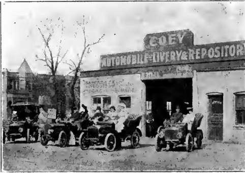
The first building erected for an Automobile Garage—built by C. A. Coey
